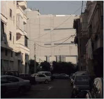
View from the alley behind the mall towards the blind wall
