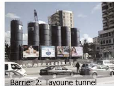
Barrier 2: Tayoune tunnel
