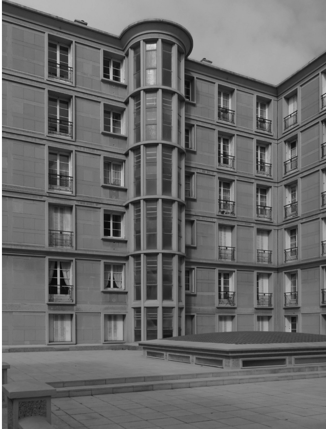
The load-bearing architecture with prefabricated infill elements. Le Havre: Auguste Perret architect.
