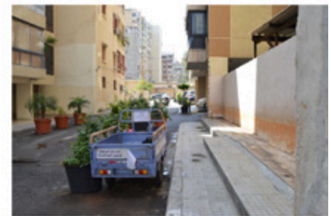
SITE B: New road between Wassef Baroudi street and Hassan Medawar. The road cuts through the existing fabric and creates without any planning of the residual left over.
